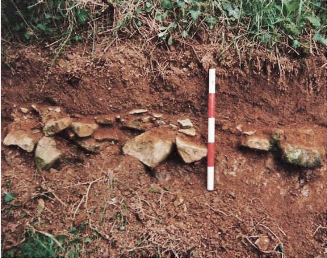
Fig. 3. Detail of the road surface (metalling) and its underlying make-up seen in section at the Den Brook exposure: 25cm scale. (photo by Pamment Salvatore 1992).
